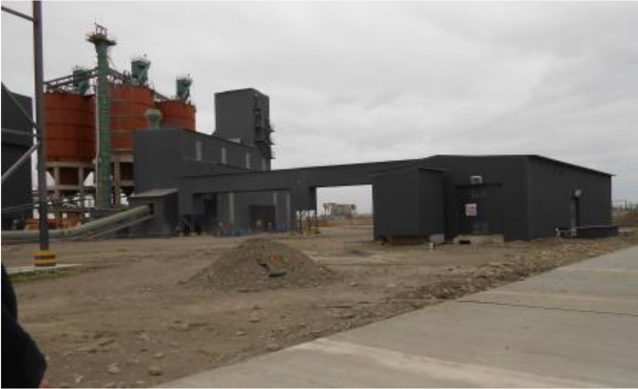
LaFarge cement plant, Poti, Georgia– 1.5 km road; year 2017.
