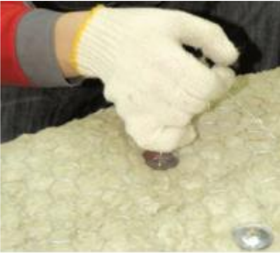
Welding of pins through insulation.
